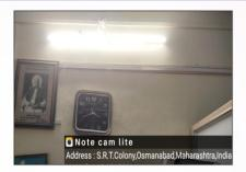
Observations: Existing lighting Tube are installed without reflectors.
